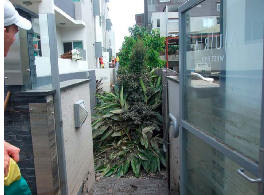
Street entrance down some steps at the side of the building leading to the fire stairs halfway along and showing the water heater room (white walls) in the middle
