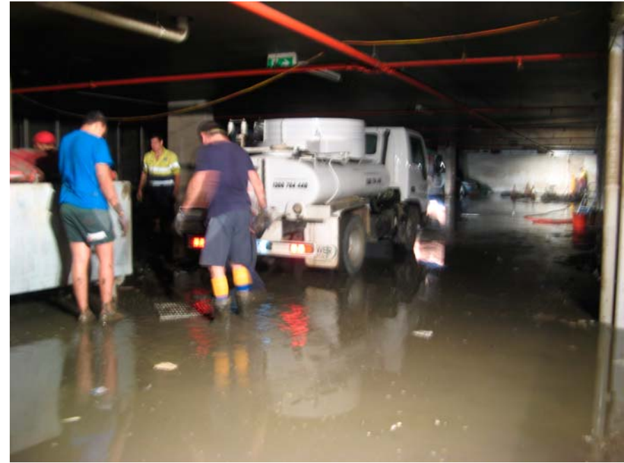
Pumping out the mud from the sump pumps on 29/01/11
