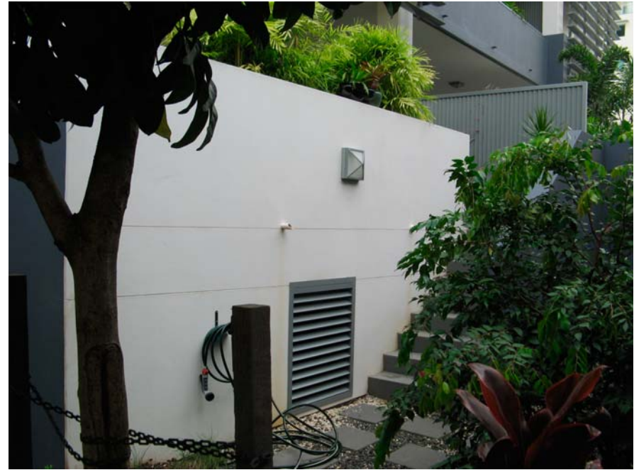
Vents at the back of Aura with the sunken garden below ground level
