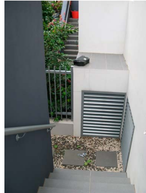
Stairs from ground floor leading to back garden with vents where water spilled into B1 carpark
