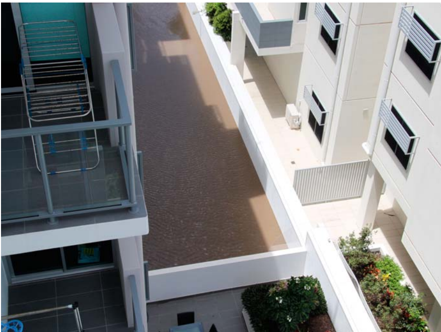
View of the carpark entrance with water still rising at 1.19 pm on 12/01/11
