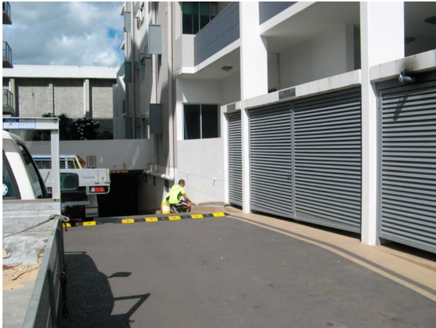
Two rooms either side of refuse room below ground floor beside the carpark entrance housing the fire sprinkler pump (left), the main fire pump and controls (right)
